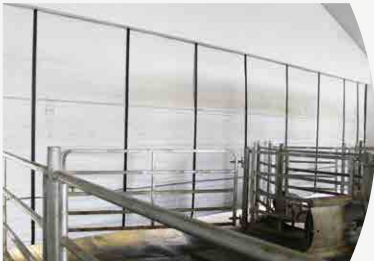
Inside Milking Parlor. Shown In Closed Position
