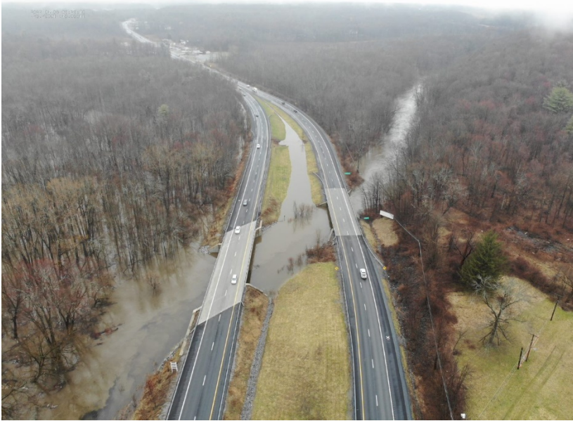
DJI_0296 - An aerial view of State Route 9 over the Kayaderosseras Creek in the City of Saratoga Springs, as seen from a Saratoga County Sheriff's Office drone. Several roadways across the county were closed due to heavy rains that impacted the region on Thursday evening, April 7 th . Do not attempt to cross flooded roadways. Turn Around Don't Drown.
