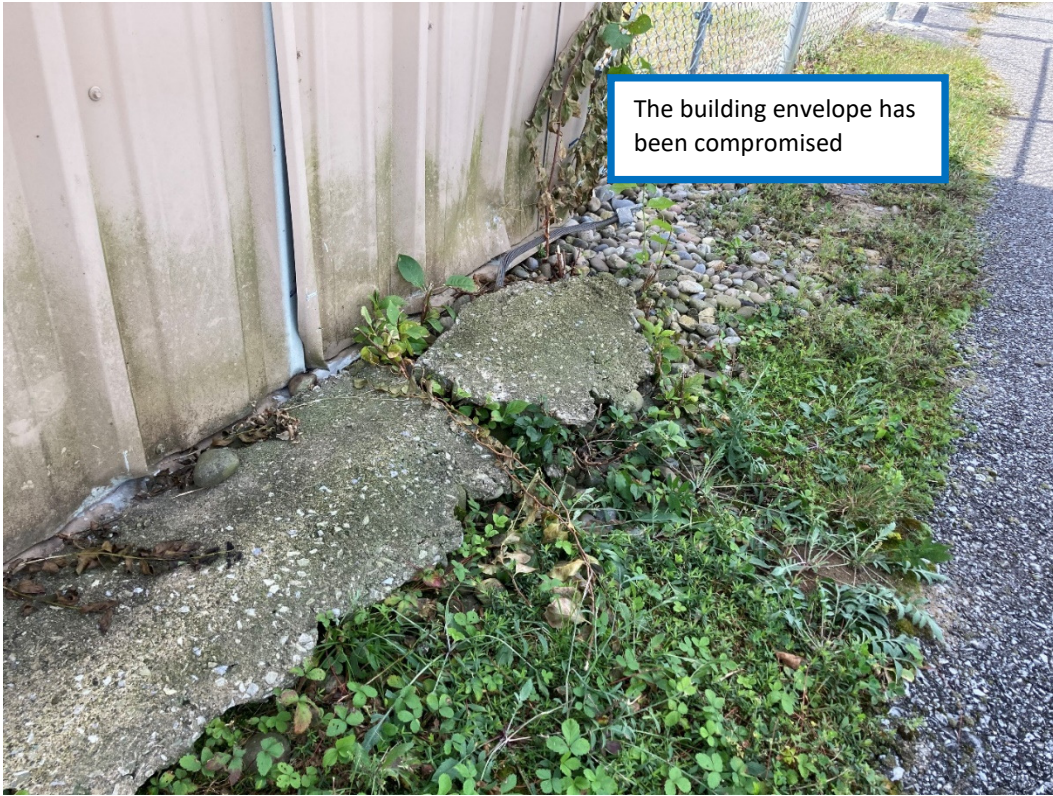
Hangar 1 Face along Main Apron
