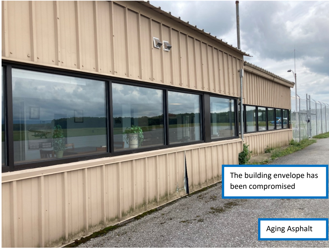
Hangar 1 Face along Main Apron
