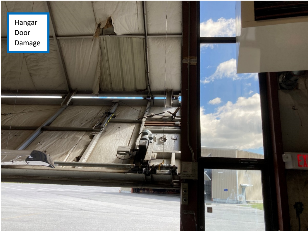
Hangar 1 Door from Inside
