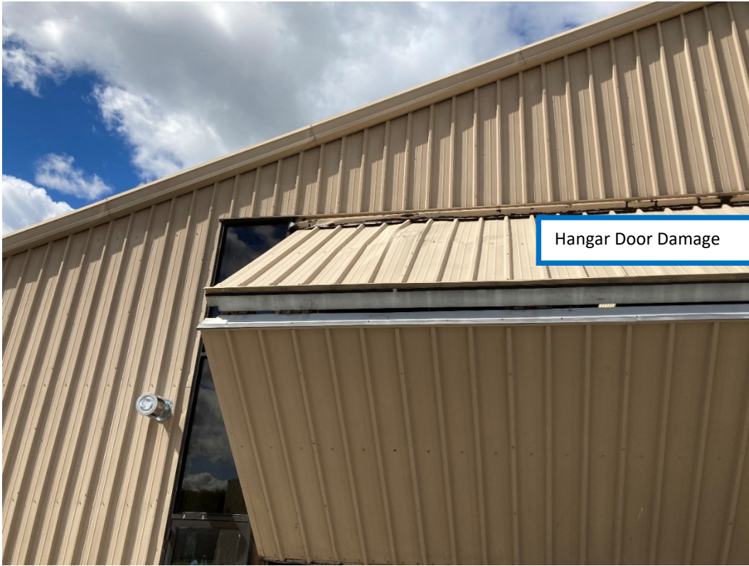
Hangar 1 Door from Outside
