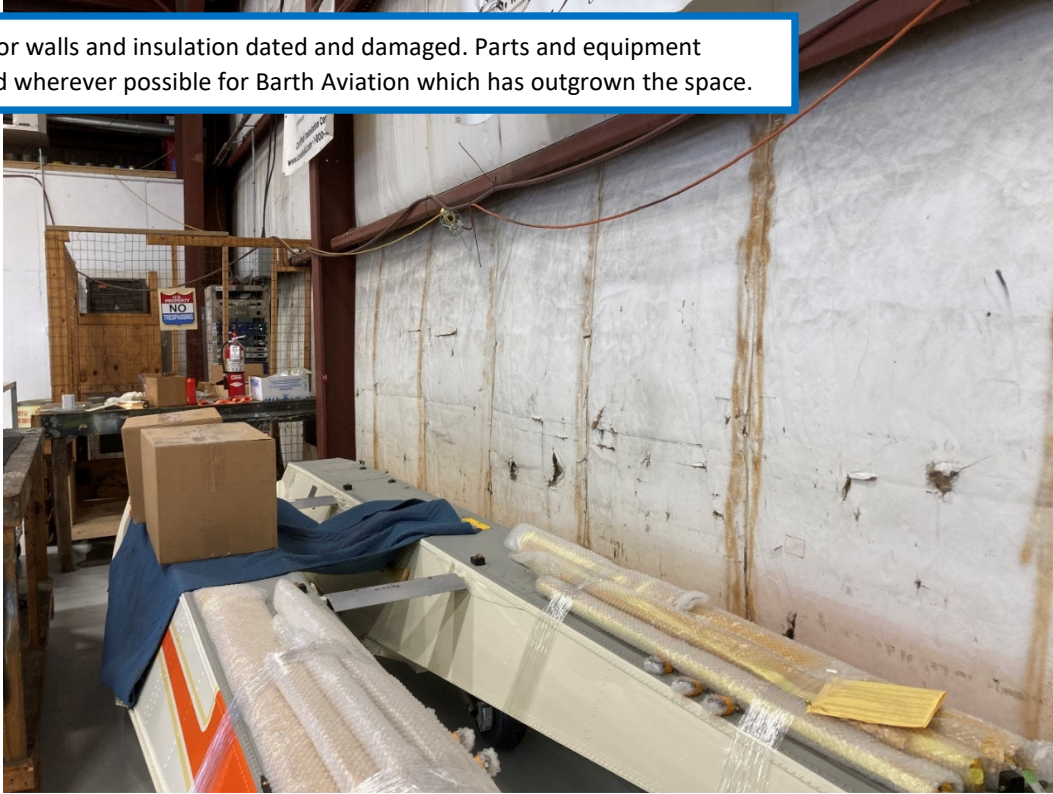
Hangar 1 interior and insulation
