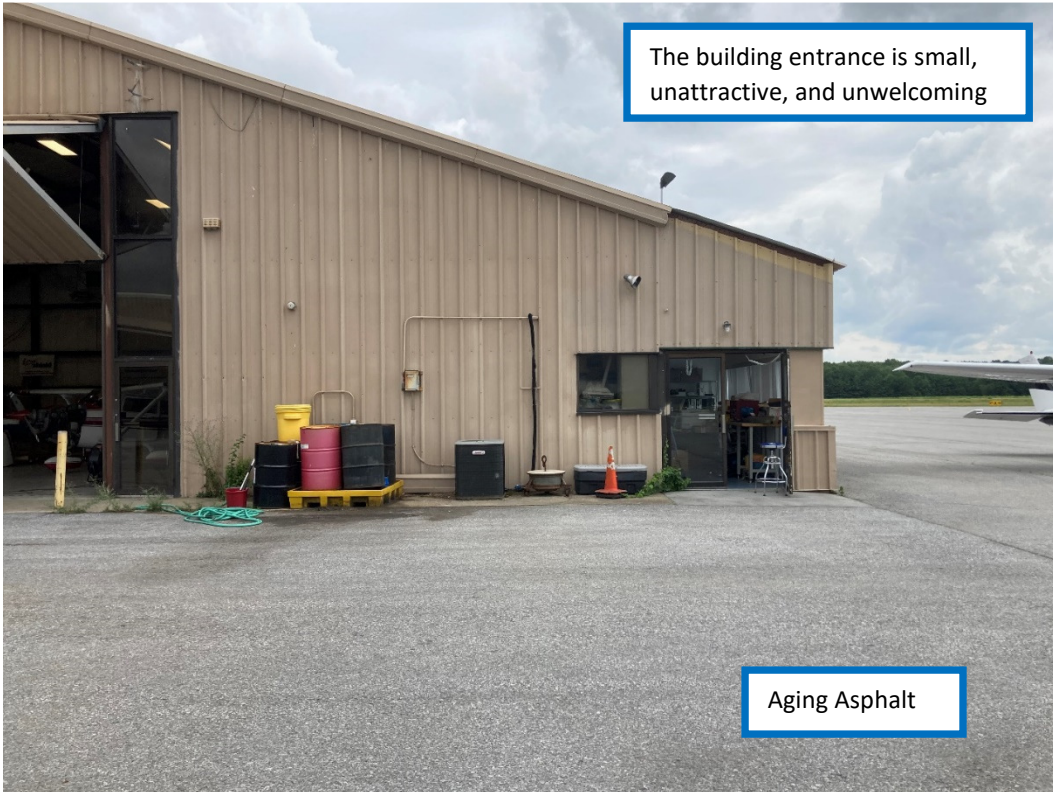
Entrance to Hangar 1 from Main Apron
