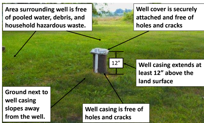
Figure 1: Photo of a properly constructed well.
