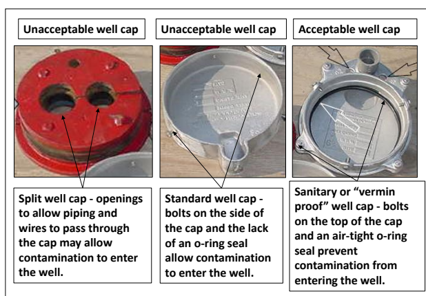
Figure 2: Photos of acceptable and unacceptable well caps
