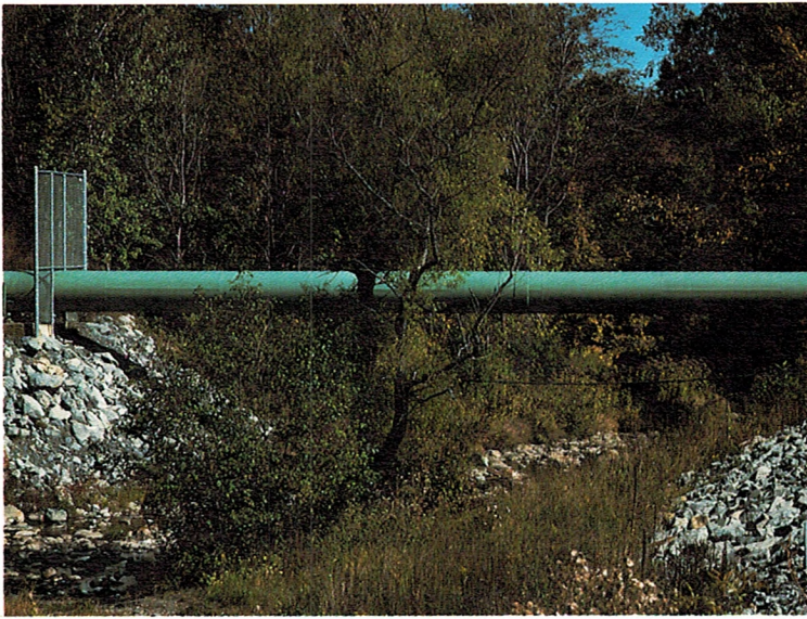
Interceptor Sewer Crossing Mourning Kill
