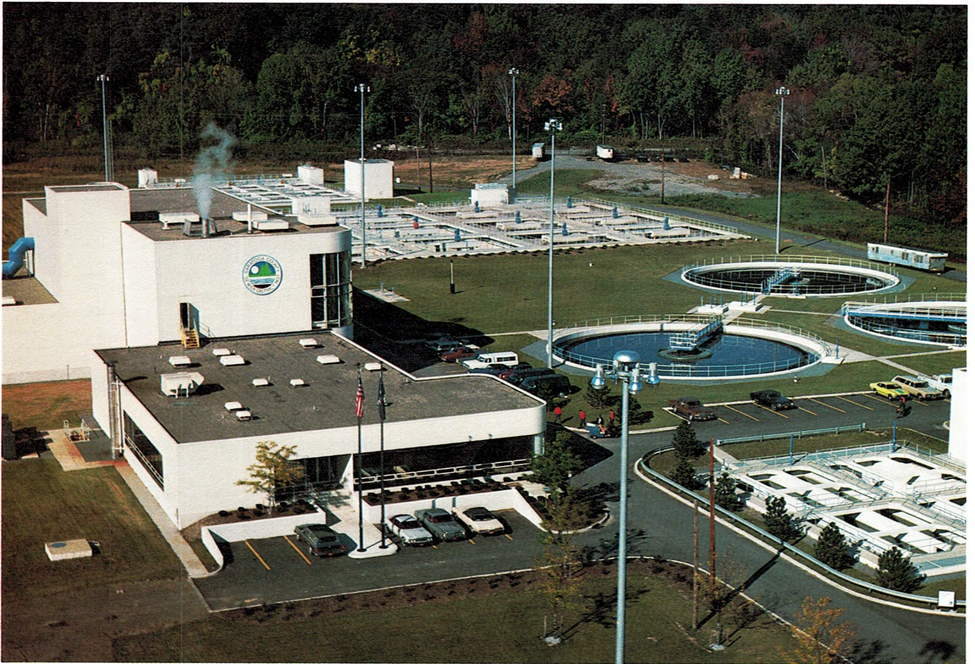
District Headquarters and Treatment Facilities
