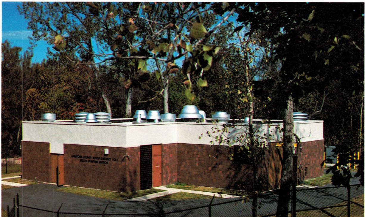
Milton Pumping Station
