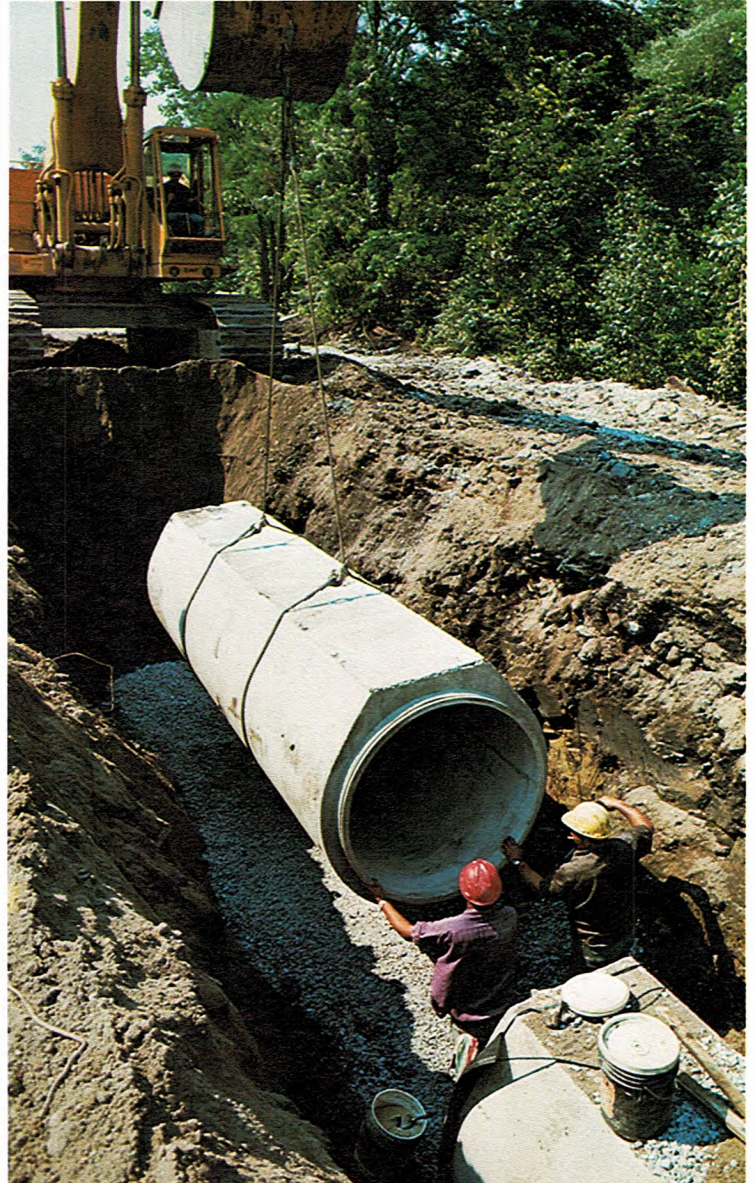
Installation of Main Interceptor Sewer through Stillwater
